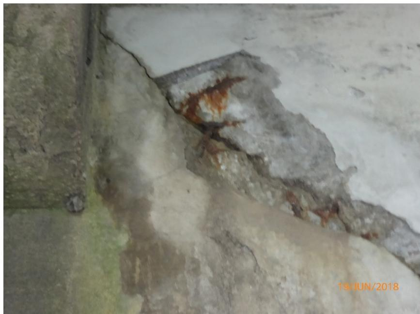
Figure 18 - Reinforcement corrosion
