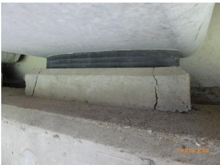
Figure 27 - Wear, mechanical2
